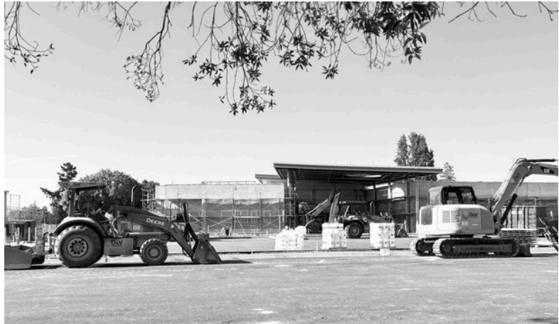
Lakewood Library getting its final shape. Photo credit: Pat
